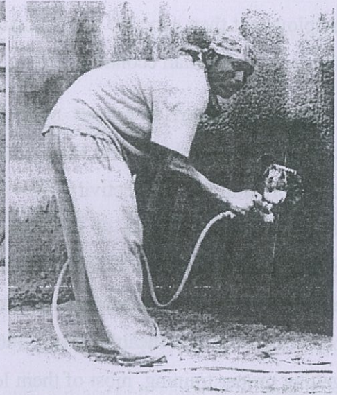
Figure 16: painting outside without proper protection
